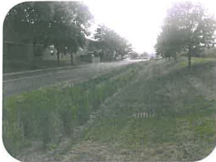
Underdrained Bioretention Swale, South Portland, Maine
